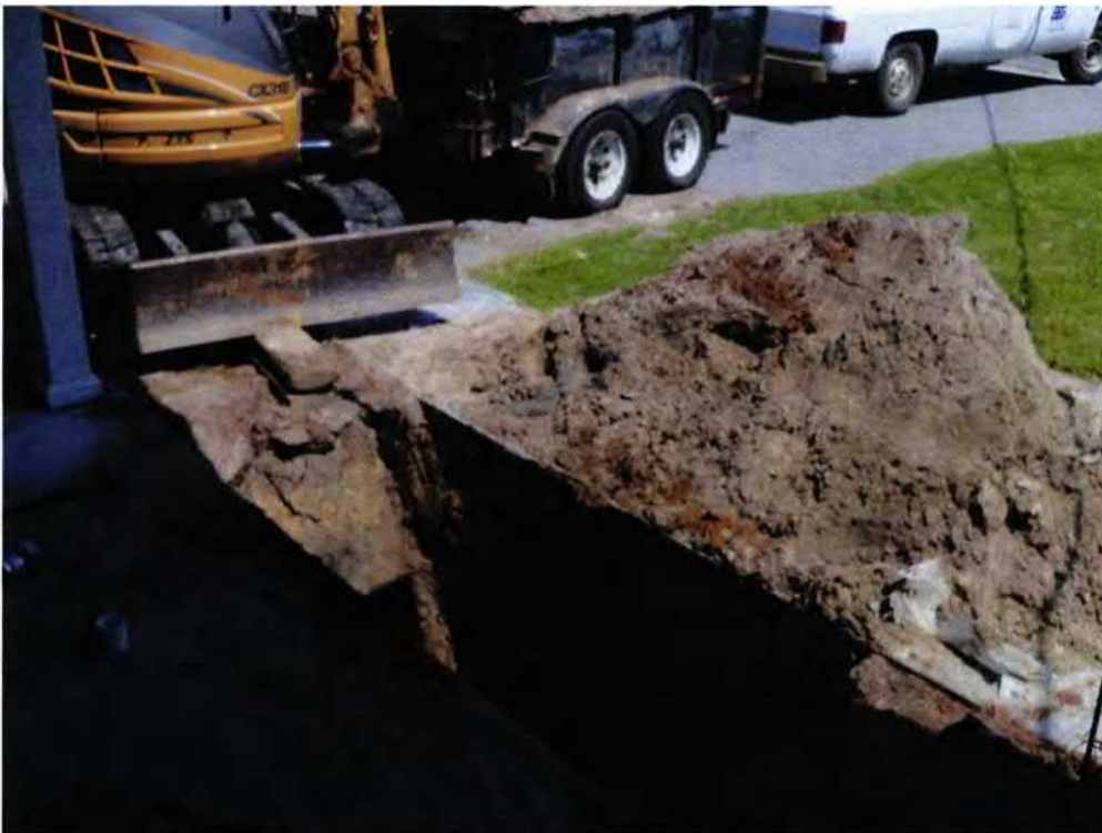
Picture 2: UST 154LaurelBB excavation in progress.
